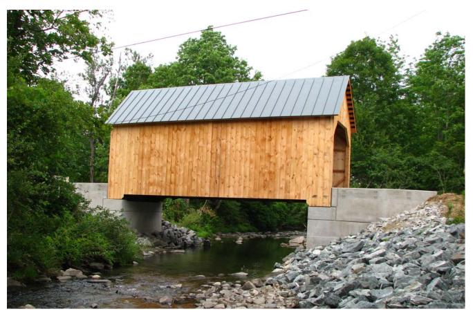
Bower's Bridge (45-14-11) in Windsor County, Vermont After being washed downstream by floodwaters in August 2011 (top) the bridge was repaired and set on new abutments on July 14, 2012 (bottom). Photos by Bill Caswell
