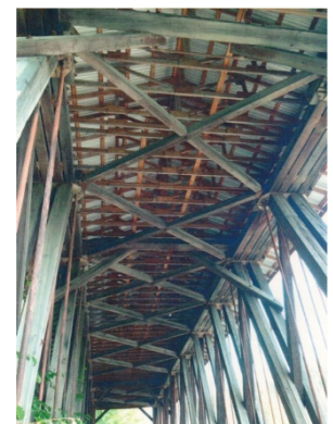
Left: Highway deck of the bridge looking north toward the Chickaloon River Right: Protective roof structure and upper diagonal truss work of the bridge July 2017 Photos by “BJ” of Palmer, AK via Ray Freden of Pembroke, ME
