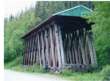
Chickaloon Railroad Bridge with added protective roof
