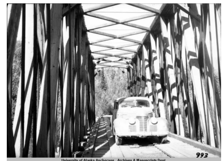
Chickaloon Railroad Bridge after conversion to a highway bridge – 1941. Russ Dow papers, Archives and Special Collections, Consortium Library, University of Alaska Anchorage
