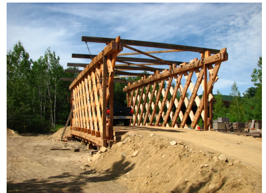
Test structure at Campton, New Hampshire.
