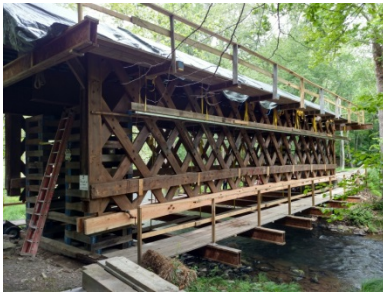
The downstream side with its new lower chord.
