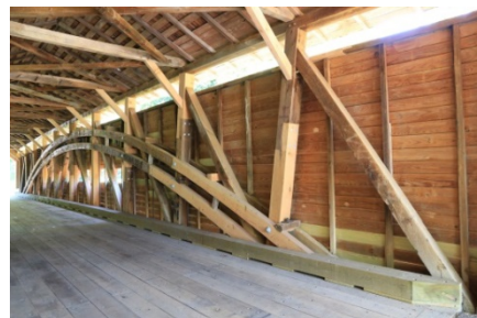
Photo of Repaired Truss by Steve Wolfhope, July 30, 2017
