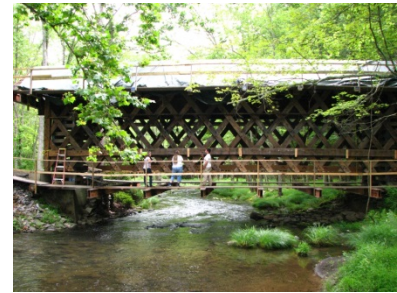
The unfinished upstream side.
