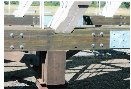
New lower chord Alan Viewig Photo August 13, 2022
