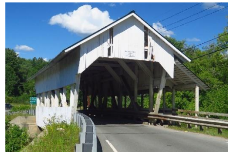
Miller's Run Bridge VT/45-03-06#2
