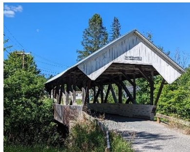
Chamberlain Mill Bridge VT/45-03-04
