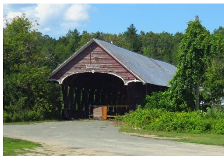
Sanborn Bridge VT/45-03-05
