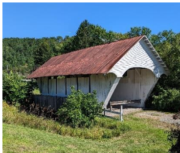
Schoolhouse Bridge VT/45-03-03
