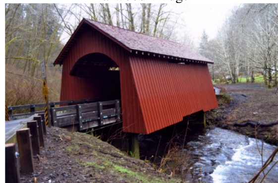
North Fork Yachats Bridge
