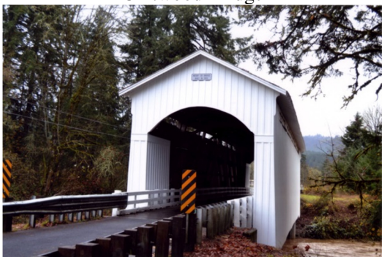
Mosby Creek Bridge
