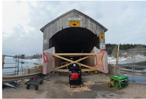
Large timber beams were inserted to support the bridge during repairs. They were also used to reinstate camber back into the structure.
