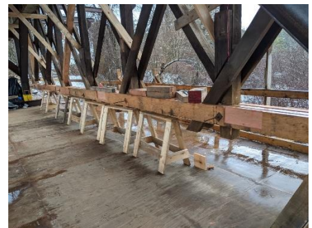
New lower chord in place.
