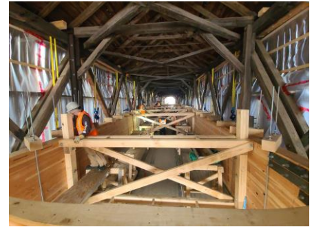
Large timber beams were inserted to support the bridge during repairs. They were also used to reinstate camber back into the structure.
