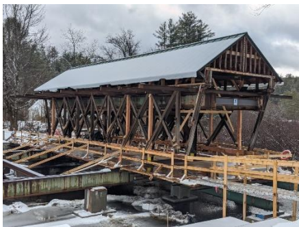
Temporarily relocated bridge.
