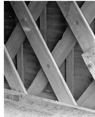
Joseph Conwill Photo of Single Pin Connection
