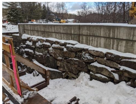
New southern abutment.
