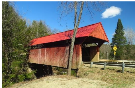
Red Bridge Franklin County VT/45-06-11
