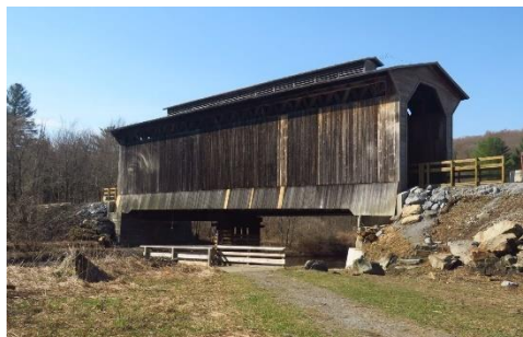
Fisher Bridge Lamoille County VT/45-08-16
