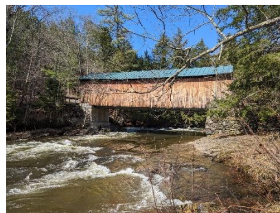
Montgomery Bridge Lamoille County VT/45-08-14
