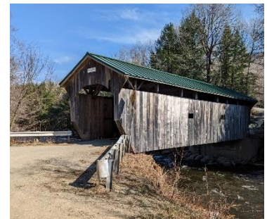
Morgan Bridge Lamoille County VT/45-08-07
