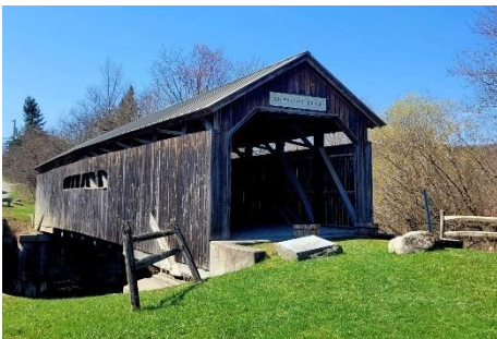
Brown River Bridge Chittendon County VT/45-04-05
