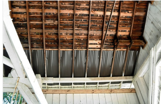
New corrugated roof sections on Gilkey Bridge
