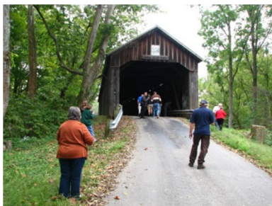
George Miller Bridge.
