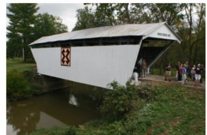
Kirker Bridge. Scott Wagner Photo
