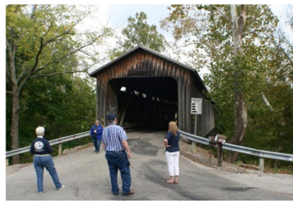
North Pole Road Bridge
