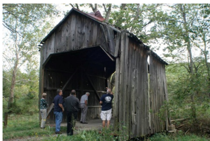
Valley Pike Bridge
