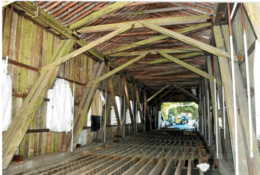
Interior of the Belknap Bridge
