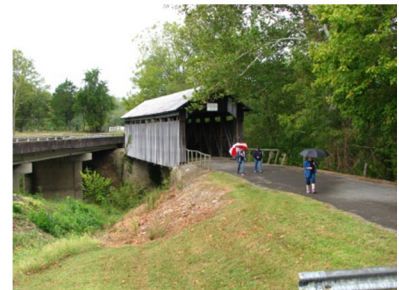
Ringos Mill Bridge
