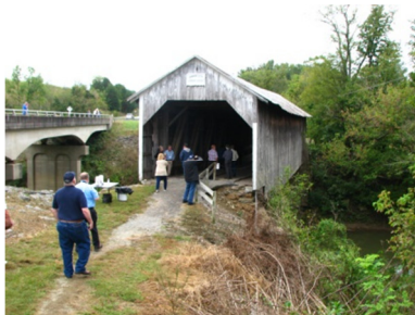
Grange City Bridge
