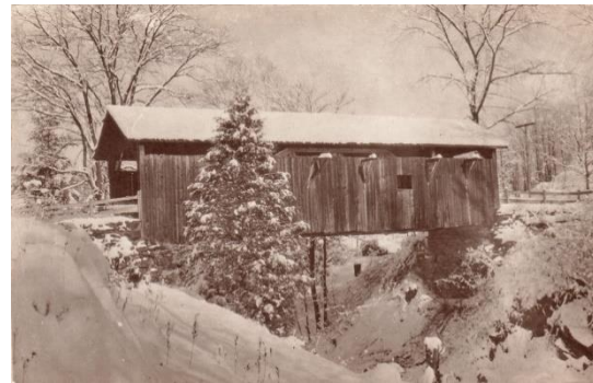
High Bridge, Waitsfield, Vermont VT/45-12-96, Todd Clark Collection
