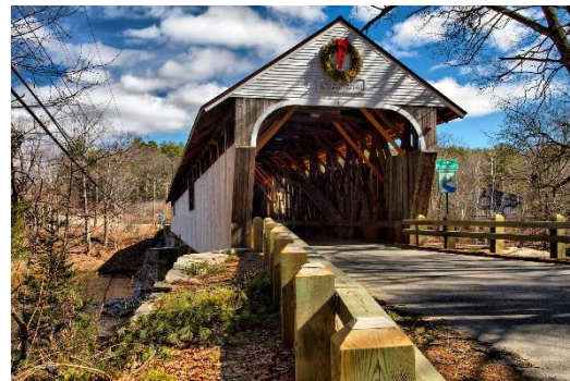
Blair Bridge, Campton, New Hampshire NH/29-05-09, Betty Pauwels Photo
