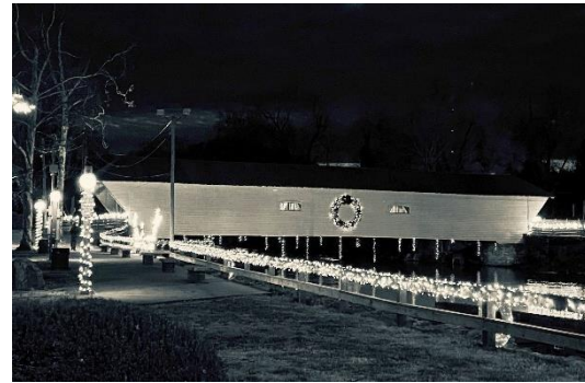
Elizabethton Bridge, Elizabethton, Tennessee, TN/42-10-01, Robert Benfield Photo
