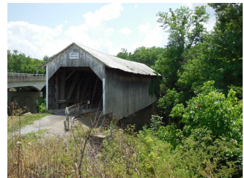
Grange City Bridge, Fleming County, KY Jim & Gloria Smedley Photo, June 2013
