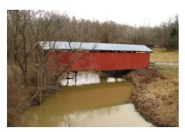
The Stevenson Road Bridge (WG #35-29-15) in Greene County is undergoing a complete renovation - truss repairs, new floor beams, flooring, roofing, siding and abutments. Work is being done b the Righter Company of Columbus, Ohio.
