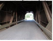
Epoxy coating added to protect the wooden deck.
