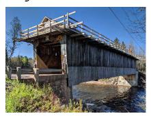
When Bill & Jenn visited the Smythe Bridge on May 25<sup>th</sup>, the roof was in the process of being replaced. When we returned during the first day of the Society's covered bridge tour on July 26<sup>th</sup>, the new roof was complete. The 139' (42 meter) single span bridge was built in 1915. (Left photo by Bill & Jenn Caswell, Right Photo by Gloria Smedley.)
