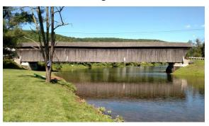
Flood waters from the East Branch of the Delaware River inundated Covered Bridge Park home of the Downsville Covered Bridge. Listed on the National Register of Historic Places, the 174-foot, single span structure includes a combination Long and Queenpost truss and was constructed in 1854. Fortunately, no damage to the bridge was reported. (April 15, 2019 article, The Daily Star.com, photo by Bill & Jenn Caswell.)
