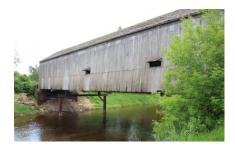
Ray Boucher, president of the Covered Bridges Conservation Association of New Brunswick reports that repairs to the Hasty Bridge near Salisbury appear to be completed. Steel I-beams have been added for additional support bringing the weight limit up from 5 tons to 10 tons. He provided these recent photos of the bridge.
