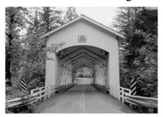
The 25<sup>th</sup> anniversary of the reconstruction of the Linn County's historic covered bridge was held this past June. The 1945 Howe truss bridge's single span stretches 105-feet across the South Santiam River and serves as the entryway into Cascadia State Park. The original bridge was constructed in 1928 and
