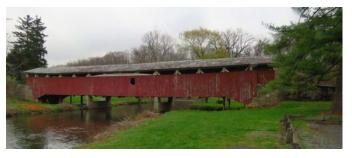
million for rehabilitation construction, nearly \$200,000 for design and more than \$150,000 for administration and inspection. The project includes repairs to the bridge railing system, approach roadway, timber deck, the superstructure, top and bottom chords, verticals, arches and the roof system. Bogert's Bridge is listed on the National Register of Historic Places. (*Photo by Bill & Jenn Caswell.*)
