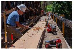
Bridgewright Tim Andrews hand chisels precision channels for truss shoes to fit into a repaired section of the lower chord. June 16, 2020.
