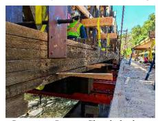
Removing Bottom Chord planks to be replaced. June 4, 2020.
