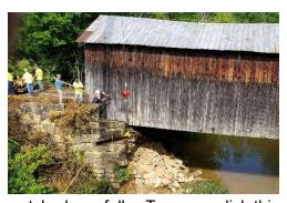
On July 1<sup>st</sup>, a steel beam was placed under the south end to prevent it from dropping any more. The beam is being held in place by a large concrete anchor. This photo shows the I-beam being moved into place by a large crane on the bridge which bypassed the covered bridge.
