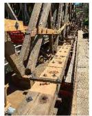
West side reconstructed chords with stitch bolts installed. June 18, 2020.
