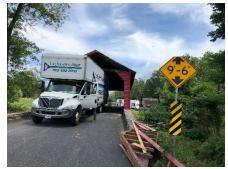
posted clearance of 9'-6". The height of the truck pushing upward on the roof structure strained a number of its connections. County officials have closed the road and bridge until repairs can be made. Amanda Radcliffe, an engineer with the county's Division of Public Works and NSPCB member, shared details and photos of the damage. Damage
