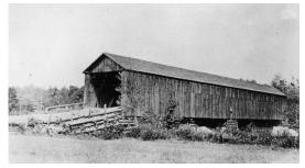
Maine DOT Photo, July 25, 1924 showing the original log-crib abutments and pier.
