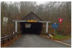
bridge was closed on June 15<sup>th</sup> to allow for some test drilling on both sides to prepare for the eventual installation of storm drain lines. Water running into the bridge from the roadway is causing deterioration of the deck boards so the county is working to alleviate that. They are also looking to improve daytime lighting
