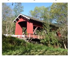
Humbolt County Board of Supervisors was scheduled to meet in December to outline the work needed to repair the Brookwood Covered Bridge (WG #05-12-02) a 66 foot, single span Howe Truss structure built in 1969 to span the Jacoby Creek. The scope of work is to include verification of the bridge's actual condition, roof and paint inspections and fumigation of the bridge.
