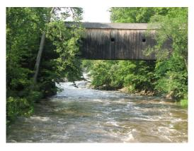
November was to see the closure of the historic Bull's Covered Bridge (WG #07-03-01) to allow for the replacement of its roof last replaced in 1994. The 109 foot, single span structure was built over the Housatonic River in 1842. The bridge incorporates an unusual Town Lattice / Queenpost / Kingpost Truss combination. The nearby West Cornwall bridge has a similar truss.
