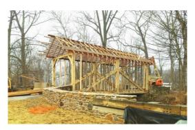
The Roddy Road Covered Bridge (WG #20-10-02) near Thurmont, Maryland was badly damaged by an oversized vehicle on June 16, 2016. Work on the bridge began in October and was nearly complete at the end of February. The large timbers are new and this will be listed as a new covered bridge.
