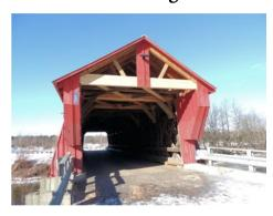
On December 15<sup>th</sup>, *Le Guide de Cowansville* reported that the covered bridge in that town was damaged that morning after being struck by an oversized vehicle. The bridge had wooden "headache bars" to alert drivers of the low clearance. Those were completely destroyed by the passing truck. The bridge is posted for 2.70 meters (8'-10") and a 3 ton weight limit.
