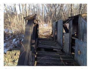
Will continued by mentioning that the overgrown status of the former road would make access to the site by fire or police vehicles very difficult. Since the bridge appears to be structurally sound, he recommended that the floor and cladding be replaced to protect the truss elements and fire retardant applied to them to provide additional protection from vandals.
