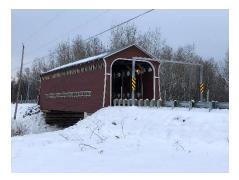
Repairs to the Pont Caron were completed in December and it is now open to traffic. A number of structural timbers were replaced and some spliced with new pieces. Headache bars have been added near the portals. The bridge, which used to be gray, has now been painted red. (*Photos by Pascal Conner.*)
