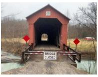
The Hune Covered Bridge, built in 1878 is again closed to traffic. A creeping landslip on the southeastern bank of the Little Muskingum River developed between January 5 and 6, following wet weather. The slip affected the Duff Road approach to the bridge. On January 7, the bridge
