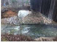
¹ **shotcrete** – concrete or mortar sprayed pneumatically at high velocity onto a surface, first used in 1914, and typically reinforced by conventional steel rods, mesh or fibers. The visible dry laid stonework façade was added here to hide some of the shotcrete providing a more natural appearance.
