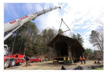
rehabilitation design work proceeded. Repairs were designed for the roof framing, upper and lower lateral bracing, timber trusses, board siding, and bearings. Both abutments are to be removed and replaced with concrete abutments and wingwalls. The east abutment will be raised 2 feet to enable greater capacity of the bridge to pass future floodwaters without damage.
