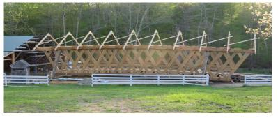
24" in length. Nineteenth century techniques were used to raise the trusses to vertical. Floor and roof trusswork are being added. When ready, the bridge will be positioned about 90-feet away at the bridge abutments on 4' diameter wooden rollers. The abutments consist of huge granite blocks, weighing about 300-tons and collected from old foundations all over Maine and New Hampshire, all fitted into place without mortar, with 4-feet of supporting stone and material beneath the water line.
