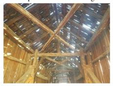
Holes in the roof allow rain to pour Broken lower chord at the west end in and accelerate deterioration of of the bridge. the truss members.
