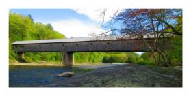
In early February, a WW Building Supply delivery truck damaged roof braces on the east side of the West Dummerston covered bridge (WG #45-13-02#2) causing an estimated \$63,000 in damages. A representative of WW Building Supply notified police of the incident and will pay for the damages. The broken trusses do not impact the capacity of the bridge so it will remain open until repair work begins.
