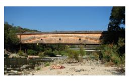
overloaded when the bridge was open to traffic. The external suspension system which was constructed to support the structure while fundraising was going on, will be removed and an existing internal steel support structure will be beefed up to provide additional support. The internal steel beams are painted a dark color and encased in wood so they do not detract from the historic scene. Finally, the bridge will get a new roof and siding.
