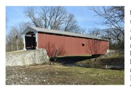
It appears that the recent work on this bridge has resulted in the majority of the truss system has been replaced with new material. Although there are no hard and fast rules about what constitutes an historic repair or replacement, we generally make that call based on whether or not at least half of the historic material is still present. That does not appear to be the case here so this will be listed as a new bridge. J. D. Eckman, Inc. was awarded the contract with their bid of
