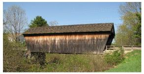
shall be expended unless such bridge may be rehabilitated to a carrying capacity of at least 6 tons". Also, truss member repairs and replacements as necessary, installing new knee braces to better brace the truss upper chord and raising the bridge by approximately 6" so stormwater drains away from the bridge deck.
