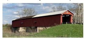
a significant portion of the metal roof that was installed when the bridge was rehabilitated in 2014. No structural damage was reported. He plans to ask contractors to replace the whole roof, as it has now come off twice in six years. He is requesting that the number of fasteners holding the metal down will be
