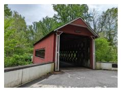
Our first covered bridge stop in Delaware was the Wooddale Bridge (DE-02-04#2). The current structure replaced a former covered bridge built in the late 1800's which was lost during flooding in 2003. The new bridge, a 60' long Town truss structure was built five feet higher above the stream. It opened to traffic on December 15, 2008.
