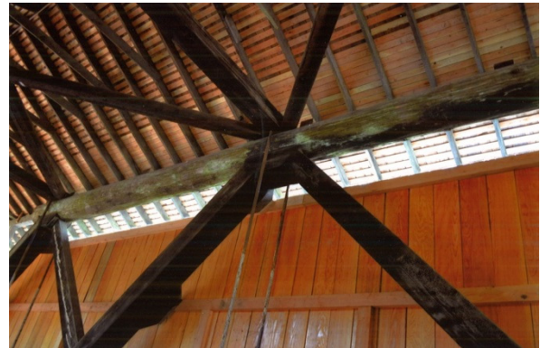
Note log used for upper chord
