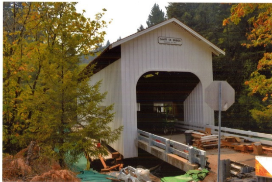
Cavitt Creek Bridge, August 2015
