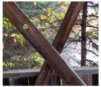
This section of the downstream truss of the Pittsburg-Clarksville Bridge is about nine inches out of alignment. Note that the trunnel which used to connect these two truss members has been sheared off.
