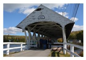
After Stark we made an unscheduled stop at the Groveton Bridge (WG #29-04-04). This 126 foot long Paddleford truss bridge was bypassed when U.S. Route 3 was reconstructed in 1939. The bridge needs some attention such as replacing missing boards and a new coat of paint. This might be a good candidate for a Society and community volunteer work day. I will contact local officials about that.
