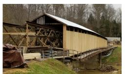
Work is nearly complete on the restoration of the Beech Fork Bridge by Arnold Grāton Associates. As of mid-November, the truss and abutment work is complete and a new metal roof has been added. Repairs have been made to the ends of the arches and new siding is being installed. Work is on track to be completed near the end of the year. (Photos courtesy Arnold Grāton Associates.)
