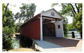
covered with stone. The lower chords and decking were replaced, and it received new
