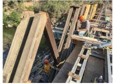
Re-installing the X-Sections of the Howe truss. September 1, 2020.
