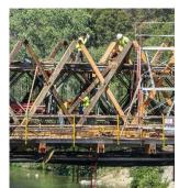
Re-installing the X-Sections of the Howe truss. September 1, 2020.
