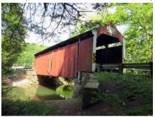
ones which only had bad sections. However, the engineering plan which we received in early October showed differently. It indicates that about 60% of the structural timbers will be replaced. They are still planning to replace a combination timber and steel floor system which was installed during earlier repairs with an all wood system. This is a
