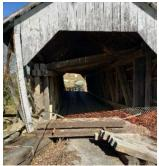
During the summer, the Grāton's and their crew inserted a steel beam under the south end of this single-span bridge built around 1867 and bypassed in 1968. The failing abutment had caused the southwest corner to drop about four feet. The beam was placed there to keep it from dropping any more until they could return in the fall to begin the process of raising it back up.
