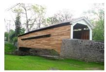
Both sides of lower siding boards of the bridge were damaged by the flooding associated with Ida. A crew from Lancaster County Timber Frames is repairing the damage. The right photo was taken after prior damage in July. *Photos by Bill Caswell and Steve Wolfhope.*
