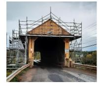
In September and October, this bridge received a new roof and siding. By the looks of the scaffolding, there may have been other work as well. The 46 meter long (151') single-span Howe truss bridge was built over Bloomfield Creek in 1918. Photos during and after repairs by Al Babineau
