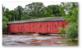
existing floor system with either a new wooden deck or a steel deck. We recommended the wooden deck option as being closer to what would have originally been constructed. They also propose to replace some of the side truss timbers which have deteriorated. We recommended that any replacements be done with wood of a similar species to what was originally used. We have also put them in contact with the staff at Wood Research and Development for additional advice on the
