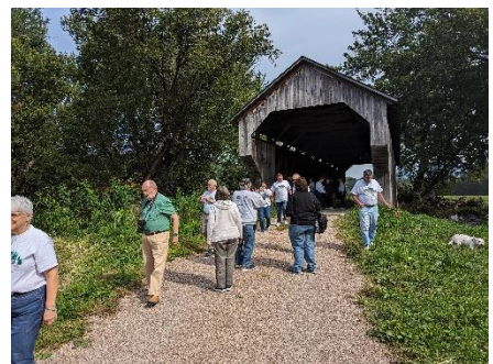
Gates Farm Bridge, Cambridge
