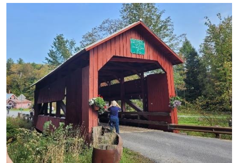
Upper Cox Bridge, Northfield Falls
