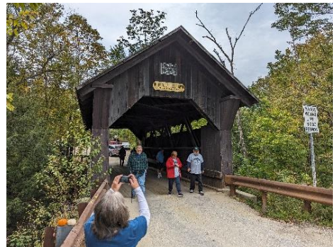
Gold Brook Bridge, Stowe
