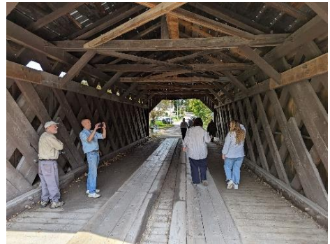
Maple Street Bridge, Fairfax
