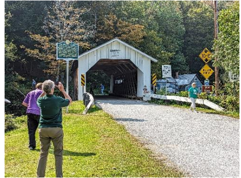
Comstock Bridge, Montgomery
