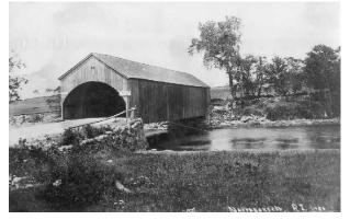
Situated at the northern edge of the village, the bridge over Narrow River was a single span Howe truss of 120', with an interesting rounded portal. It was built at a cost of \$4,834.35 and stood at this location until the road was realigned in 1920. It was replaced by the concrete Governor Sprague Bridge which itself was retired a few years ago.
