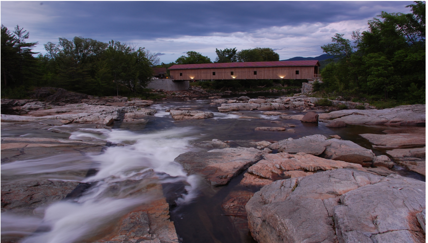
New York's Jay Bridge 175 ft. Howe Truss built in 1857 over the Ausable River (East Branch)
