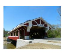
A new covered bridge has been constructed in Preble County, Ohio, to add to the seven historic covered bridges within the county. The Preble County Engineer's Office replaced the structurally deficient, functionally obsolete steel truss bridge on Camden College Corner Road over Four Mile Creek erected in the 1920s. Hueston Woods Covered Bridge is a single
