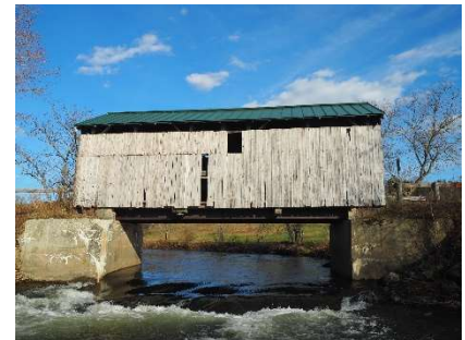
Scribner Bridge Lamoille County VT/45-08-09 Photo by Philip Caston
