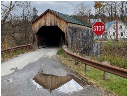
East Fairfield Bridge Franklin County VT/45-06-03 Photo by Gloria Smedley
