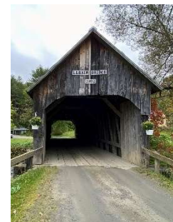
Larkin Bridge Orange County VT/45-09-10 Photo by Todd Clark
