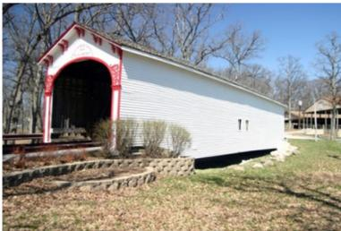
The roof will be replaced, along with the siding. The bridge will be repainted and minor asphalt and concrete work will be completed to the decking as well. Workers will attempt to reuse as much of the original wood as possible during the restoration. The intent is to be able to open it to light traffic such as Crown Point's Molly the Trolley. The project is expected to take three to four months to complete.
