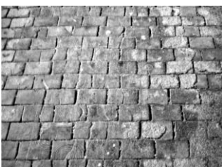
Wooden block floor. Photo by Greg McDuffee
