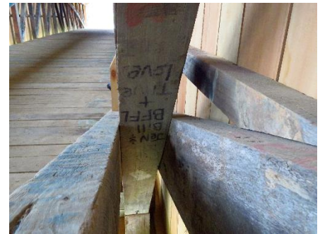
“Jen & Bill” timber after restoration
