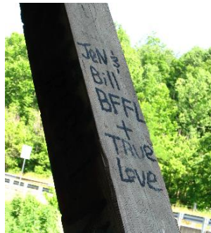
“Jen & Bill” timber before restoration
