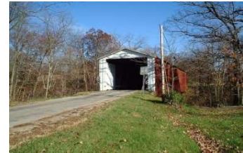
Rob Roy Bridge
