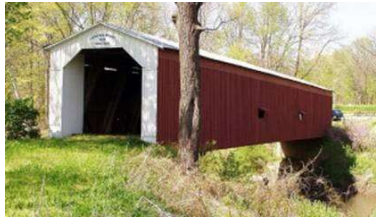
Cades Mill Bridge
