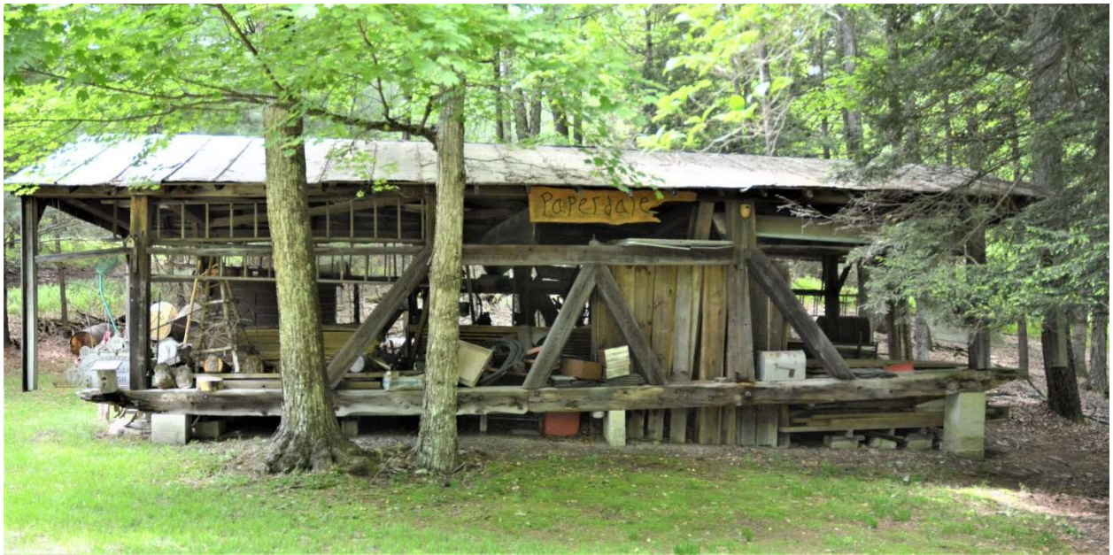
McHenry' Mill/Paperdale Covered Bridge #38-19-46
