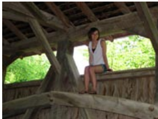
Old Keefer's Mill Bridge
