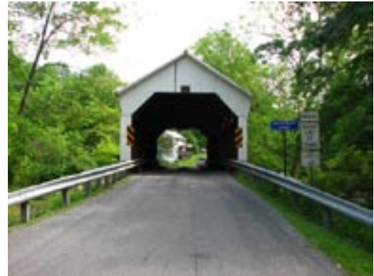
Factory or Horsham Bridge
