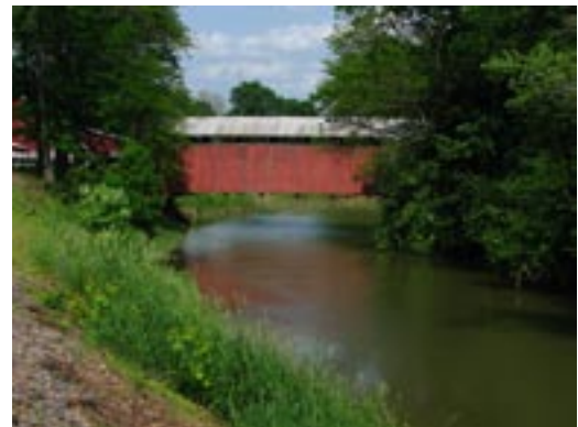
Sam Wagner Bridge
