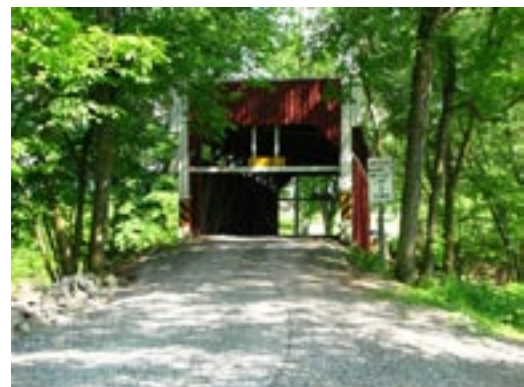
Old Keefer's Mill Bridge
