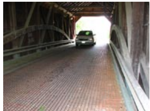
Interior of the Hassenplug Bridge
