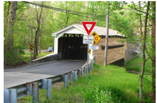
PennDOT's contractor, Eastern Highway Specialists, Inc. of Wilmington, Del., will work the next two months to repair the damaged Burr Arch truss, install new ceiling joists and braces, and replace wooden cross members on the roof. PennDOT hopes to reopen the bridge by mid-October, although the work is weather-dependent.
