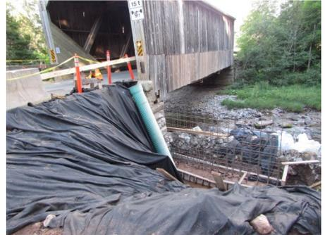
New wing wall being constructed.
