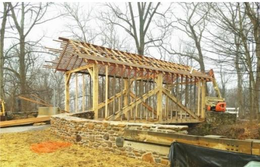
The Roddy Road Covered Bridge (WG #20-10-02) near Thurmont, Maryland was badly damaged by an oversized vehicle on June 16, 2016. Work on the bridge began in October and was nearly complete at the end of February. The large timbers are new and this will be listed as a new covered bridge.
