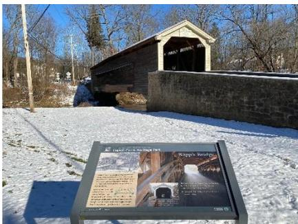
In the last issue we noted that a crew from Lancaster County Timber Frames was repairing the damage caused by Tropical Storm Ida in early September. Jim & Gloria Smedley visited the bridge on January 8<sup>th</sup> and found that it was repaired and open to traffic. The single-span Burr truss bridge was built in 1866. *Photos by Gloria Smedley.*
