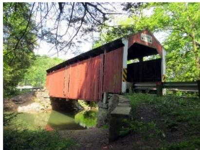
which lists the needs of the structure and desired repairs. After reviewing the document, we were pleased to see that PennDOT has given serious consideration to the historic significance of the structure. While some of the timbers are significantly damaged and must be replaced, there are plans to splice new material into timbers which are only partially
