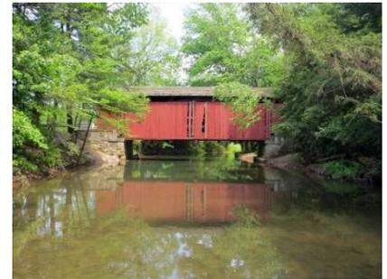
damaged. A combination timber and steel floor system which was installed during earlier repairs is intended to be removed and replaced with an all wood system. This is a welcome change from the more common plan to replace floor systems with steel beams. The Society supports the project as it is documented and we hope that it is actually repaired according to this plan. *Photos by Tim McLaughlin.*
