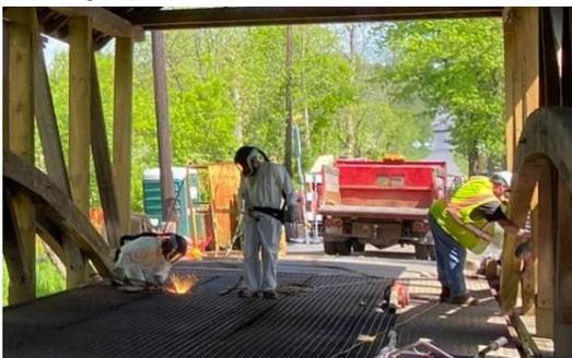
Workers also appeared to be cutting out the metal grated floor which we have heard is to be replaced with a wooden deck. The 70-foot-long span that was reportedly built circa 1825. Lancaster County Timber Frames of York, Pennsylvania, is doing the timber repairs.
