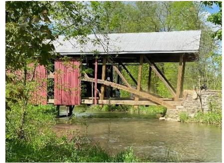
Workers also appeared to be cutting out the metal grated floor which we have heard is to be replaced with a wooden deck. The 70-foot-long span that was reportedly built circa 1825. Lancaster County Timber Frames of York, Pennsylvania, is doing the timber repairs.
