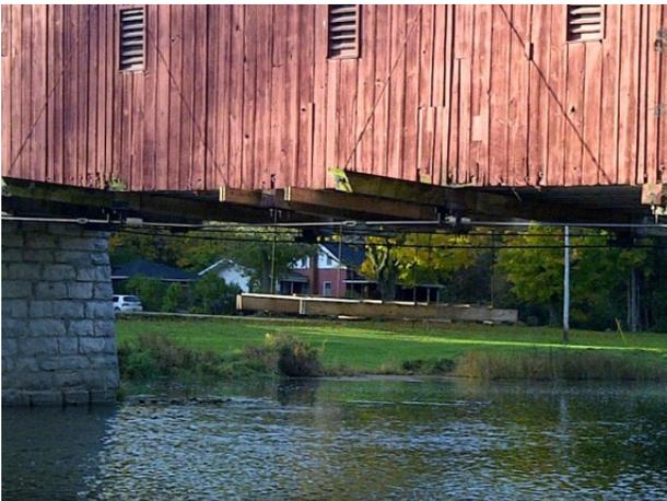
The contractor ran steel beams across the bridge, supported by a steel Bailey bridge which had been built into the walls decades ago to share the weight with the original wooden structure. Two temporary cross beams, one on either side of the damaged beam, were installed to take the load off of it.
