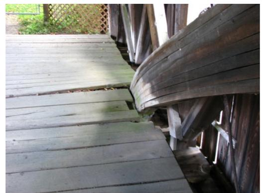
*Note the warping of the floor due to truss deformation.*
