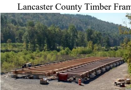
Lancaster County Timber Frames has been carving the bridge timbers for the new Blenheim Bridge in its York, Pennsylvania, shop and delivering them to the banks of the Schoharie Creek. 3G Construction of New Hampshire will assemble the bridge on the banks and move it – whole – into position over the creek. Economy Paving Company, Inc. of New York is the general contractor
