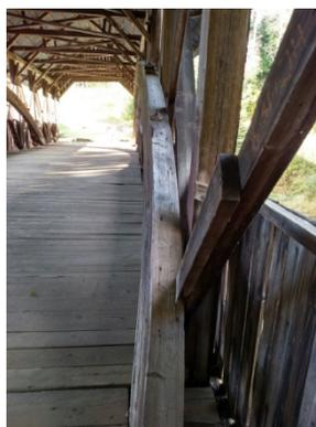
*Note the bend in the upstream truss.*
