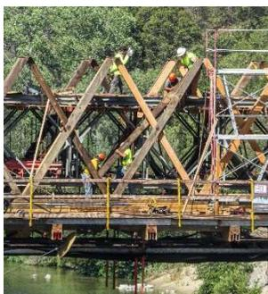
*Re-installing the X-Sections of the Howe truss. September 1, 2020.*
