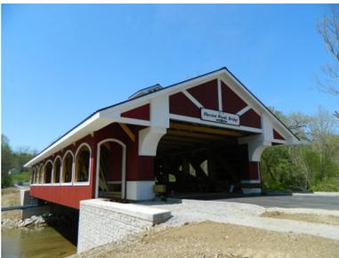
A new covered bridge has been constructed in Preble County, Ohio, to add to the seven historic covered bridges within the county. The Preble County Engineer's Office replaced the structurally deficient, functionally obsolete steel truss bridge on Camden College Corner Road over Four Mile Creek erected in the 1920s. The Hueston Woods Covered Bridge is a single span modified Burr Arch design, covered timber structure with reinforced
